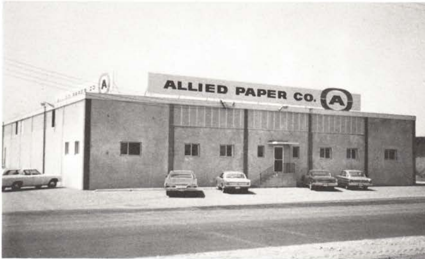
NEW WAREHOUSE - office building of Allied Paper Company, Tacoma, Washington. The structure contains 27,500 square feet of paper storage space and is located in a 100-acre industrial area.
